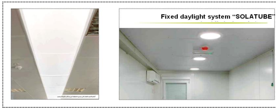
Figure (12): Using natural lighting to illuminate the interior spaces in masdar buildings in order to save energy (Source: ref. [20]).
