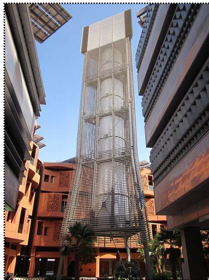
Figure (24): Use of wind towers to ventilate the squares in Masdar City
