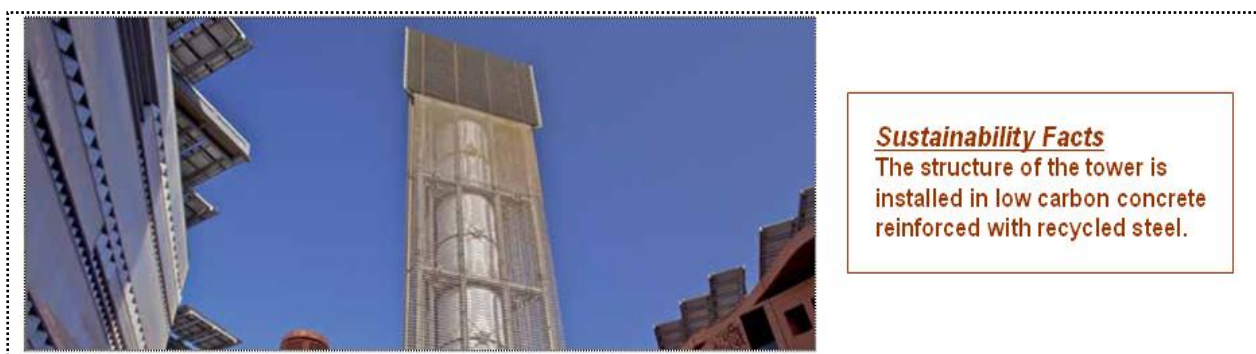
Figure (23): Wind towers in public squares in Masdar (Source: ref. [22]).
