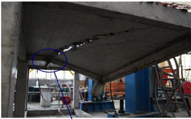
(a) Experimental Cracks for Slabs [21]
