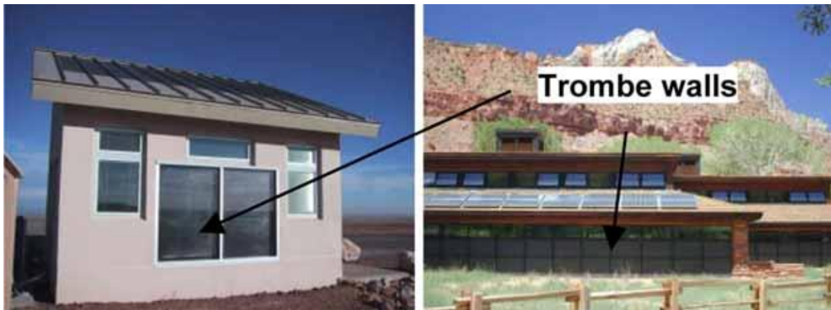
(Fig.9) Trombe Walls concept
